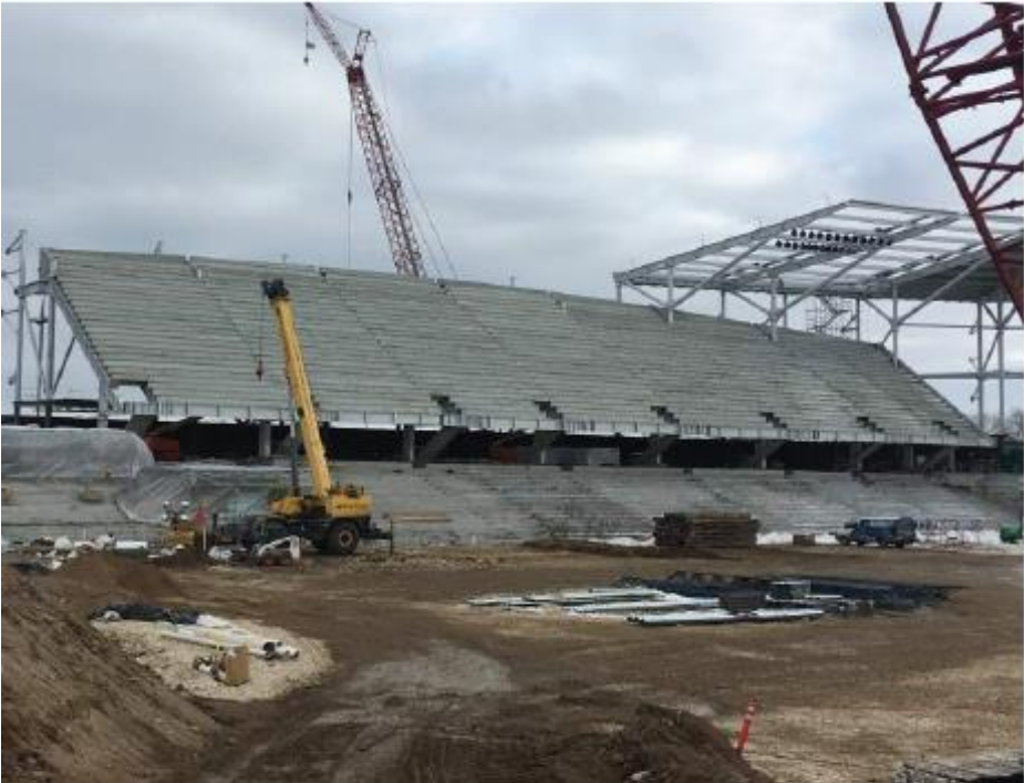
Precast Stadia Installed East Side
