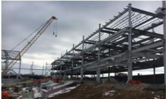
Club & Suite Level Structure
