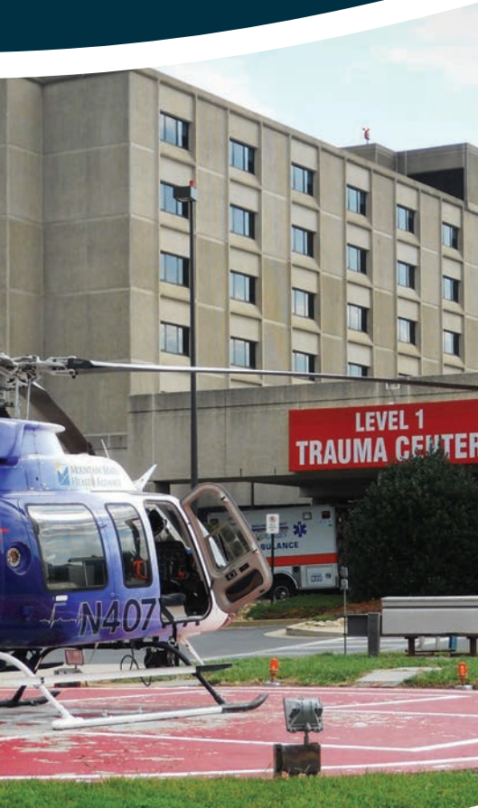
Johnson City Medical Center, TN
